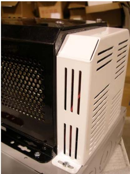
If the E-Panel kit was supplied with a DC end cover, install it using two 10-32 x 5/16" taptite screws.
